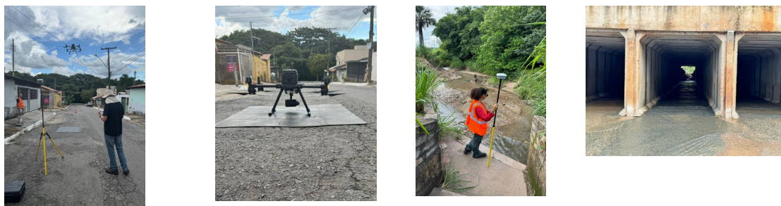
Figure 1 – Equipment used (drone) and devices surveyed in the diagnosis (Source: PDDU, 2024)
